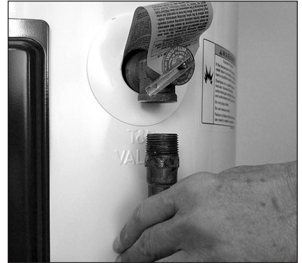
Figure 12 - Removing the T&P Relief Valve discharge pipe.
