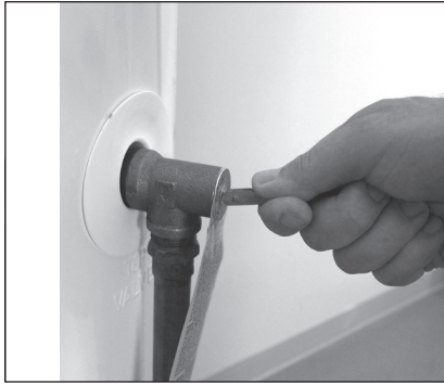
Figure 48 - T&P Relief Valve.
