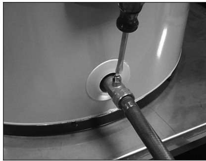
Figure 11 - Draining the old water heater.
