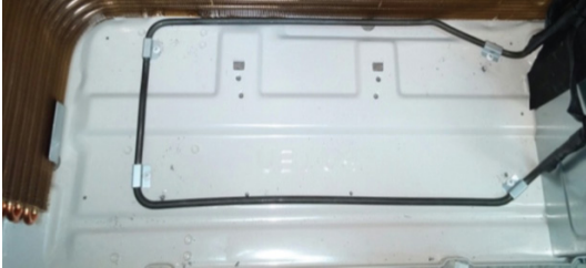
Figure 6: Outdoor Unit Drain Pan Heater.
