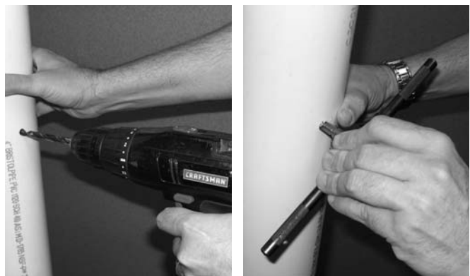
Figure 9.1: Drill and Tap Combustion Test Port
