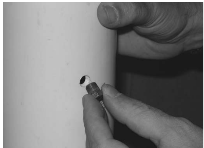
Figure 9.3: Insert Pipe Plug into Test Port
