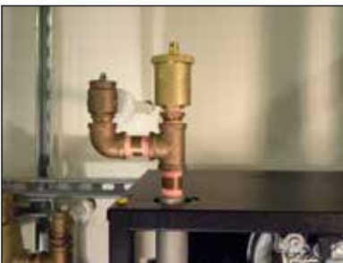
Relief valve and air vent assembly (recommended configuration)
