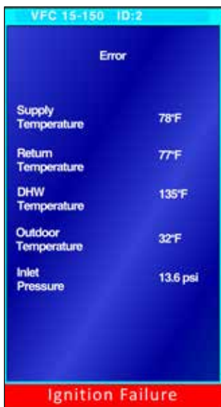
Error displayed after testing ignition safety shut off
