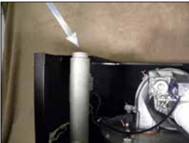
Supply stack upper tapping - 3/4" FIP to accept relief valve and air vent assembly
