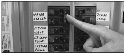
Figure 35 - Circuit Breaker.
