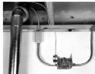
CK-63 remote mounted. For use with 120 VAC oil-fired systems. Electronic post purge is included (shown with cover off).
