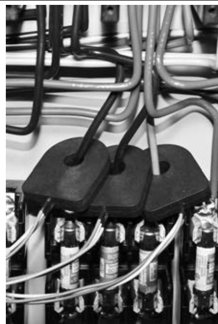
Figure 25. Heating Element Wire Routing
