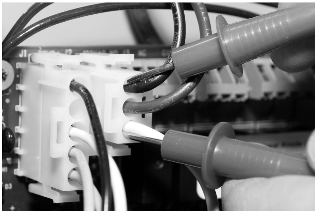
Figure 47. Checking for 120 VAC Power
