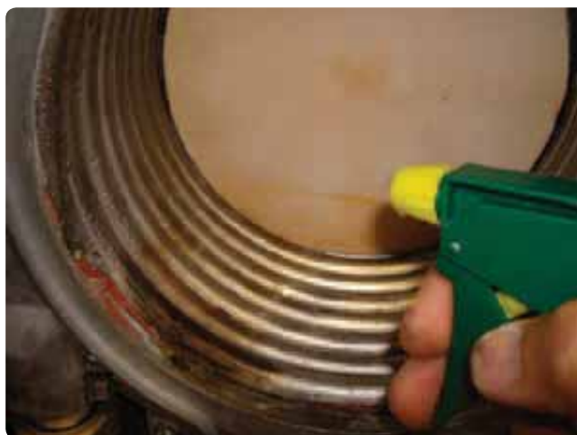
Figure 115 Cleaning the heat exchanger
