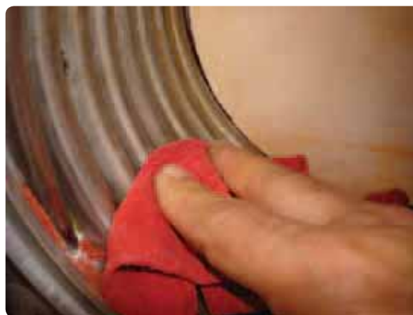
Figure 117 Cleaning the heat exchanger
