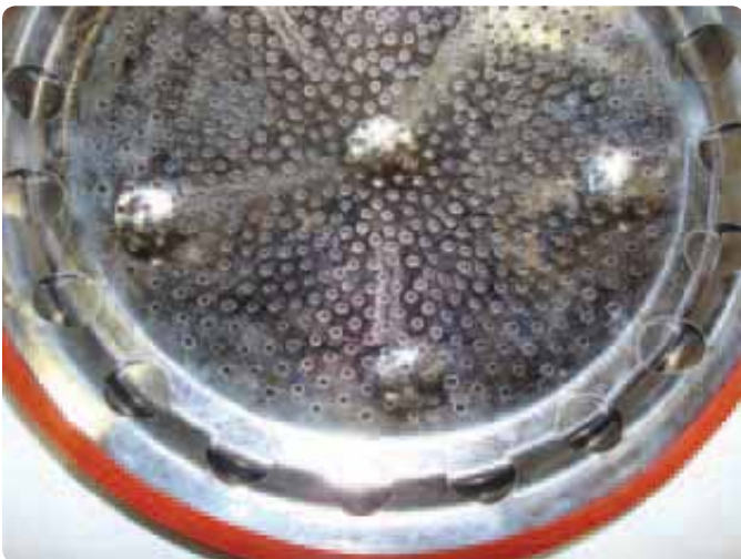
Figure 112 Inspecting interior and cleaning the burner
