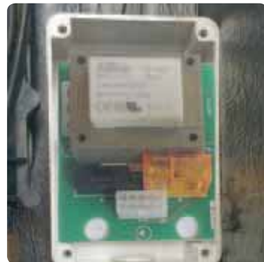
Figure 60 Thermostat-Relay box terminals Combi boiler
