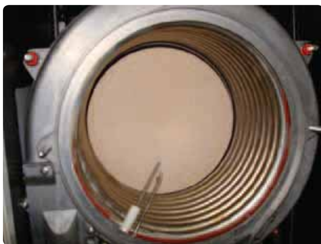
Figure 114 Inspecting and cleaning heat exchanger
