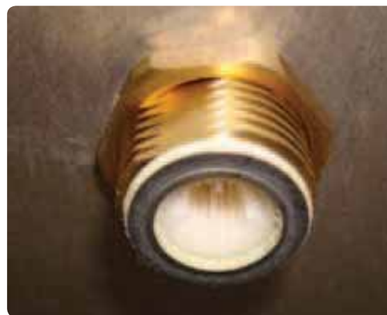
Figure 43 DHW inlet has a filter screen
