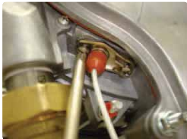
Figure 107 Removal of Ignition electrode
