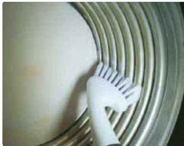
Figure 116 Cleaning the heat exchanger
