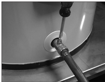
Figure 11 - Draining the old water heater.
