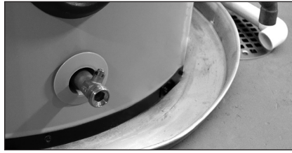
Figure 7 - A suitable drain pan piped to an adequate drain can help protect flooring from leaks and drips.
