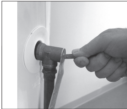
Figure 48 - T&P Relief Valve.
